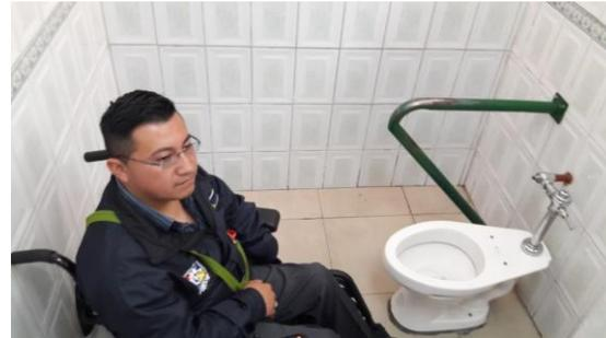
ESPACIO INTERIOR PARA TRANSFERENCIA Y USO EN CABINAS ADAPTADAS INFERIOR A 1500mm
